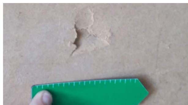
📋 Wood internal protections: Small impacts
