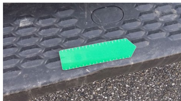
📋 Rear Step Slight deformation
