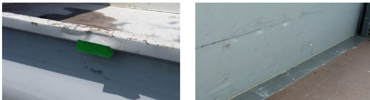
Faint scratches, Dropside/ Tipper Bodies deformations with a repair time \leq 1 h
